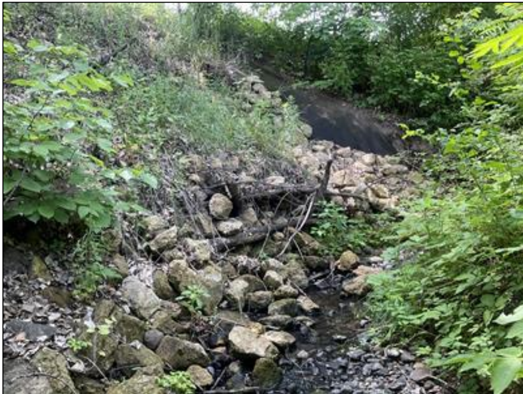
Photo 15: Severe Erosion on Middle Wentworth Creek with Evidence of Past Stabilization Efforts (Riprap over Blanket)
