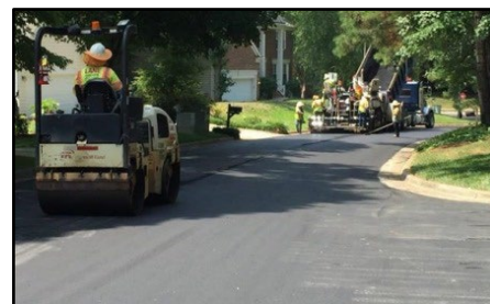
Resurfacing Asphalt (below)
