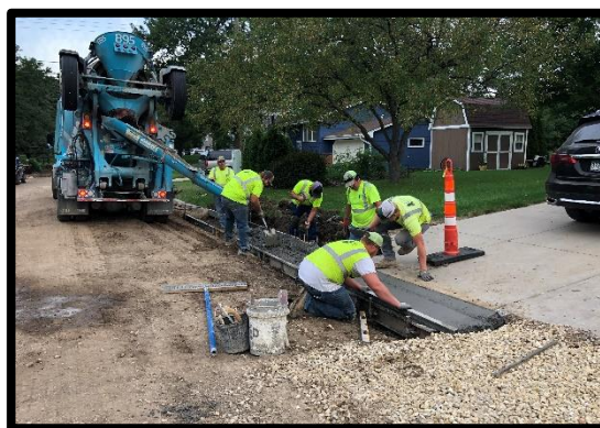
Figure 5: Spot curb replacement (City of Mendota Heights Ivy Falls Project 2021)
