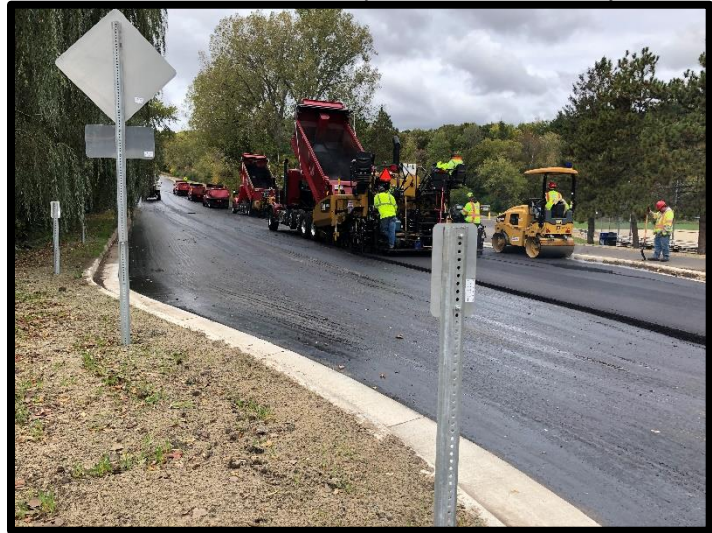
Figure 3: Reclaim and curb replacement (City of Mendota Heights Marie Avenue Project 2020)
