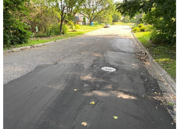
Figure 6: Roadway low point along Sylvandale Road with patching
