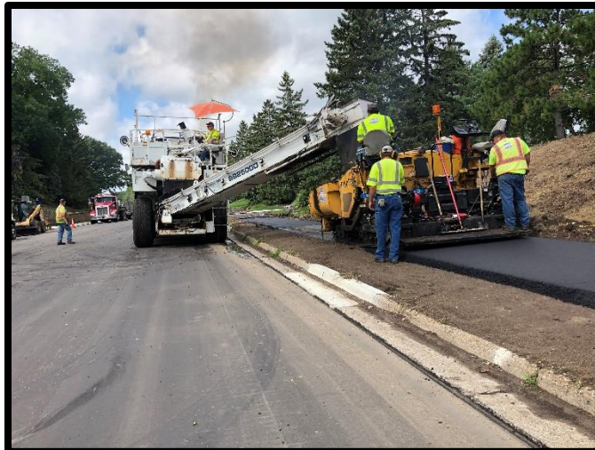
Figure 4: Reclaim and curb replacement (City of Mendota Heights Marie Avenue Project 2020)
